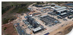
Kenya Water Treatment Plant
