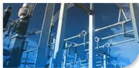
Richmond Terminal Station Rebuild
