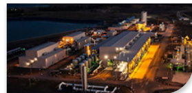
Northern Water Treatment Plant
