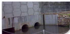
Revesby Turnback Project
