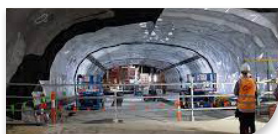
Melbourne Metro Tunnel
