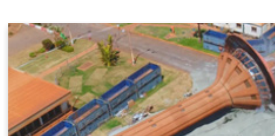
Port Headland Marine Demolition
