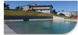
Bootawarra Water Treatment Plant
