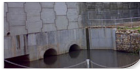
Revesby Turnback Project
