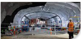
Melbourne Metro Tunnel
