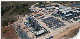
Kenya Water Treatment Plant
