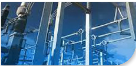
Richmond Terminal Station Rebuild
