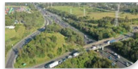
Prospect Highway Upgrade
