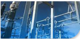
Richmond Terminal Station Rebuild
