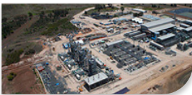
Kenya Water Treatment Plant
