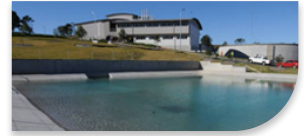
Bootawa Water Treatment Plant
