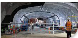
Melbourne Metro Tunnel
