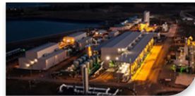
Northern Water Treatment Plant
