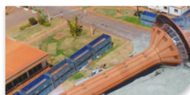
Port Headland Marine Demolition
