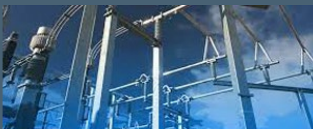
Richmond Terminal Station Rebuild
