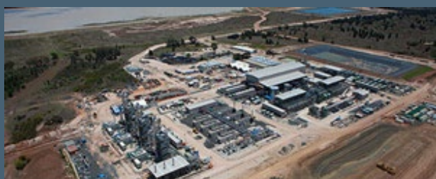
Kenya Water Treatment Plant
