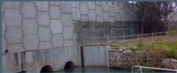
Revesby Turnback Project
